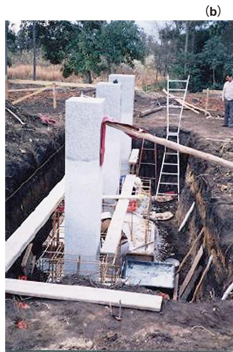
Fig. 6 (a) Area of ground excavated for installation of pillars of the absolute observation house (shaded area). Excavated to a depth of 2.0 m. (b) Photo: Installation of the pillars; Looking west from the east end.
