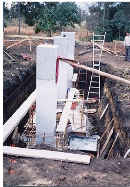
Fig. 6 (a) Area of ground excavated for installation of pillars of the absolute observation house (shaded area). Excavated to a depth of 2.0 m. (b) Photo: Installation of the pillars; Looking west from the east end.
